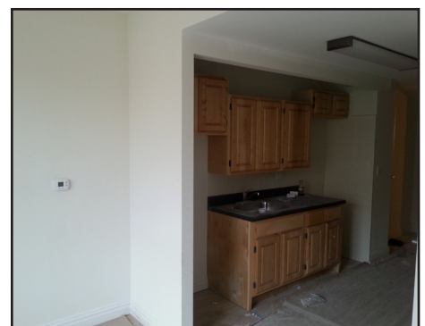
Interior shots of the apartments being constructed.
